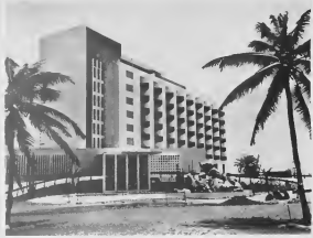
FRAMED BY picturesque palms, the new Aruba Caribbean Hotel rises above the white sands of Palm Beach. July 18, the hotel complete with 120 rooms and lavish accessories keyed to attract tourists is officially opened.
